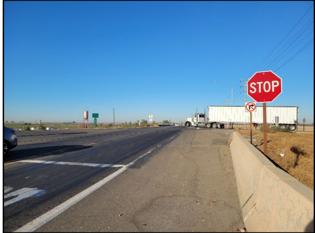
Poor lines of sight at existing northbound off-ramp
