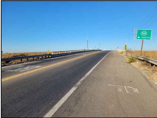
Caldwell Ave (Ave 280) Bridge over SR99
